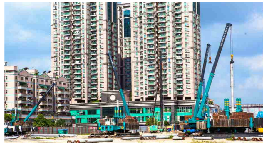
Construction of Guangzhou Huixing Business Center
