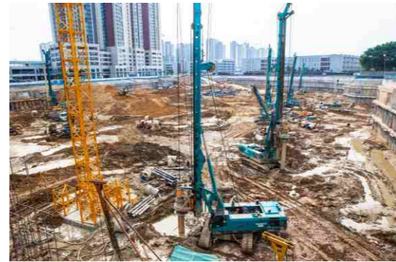
Construction in Shenzhen
