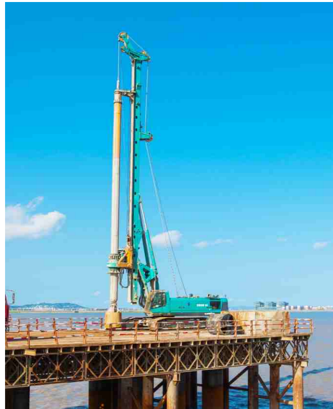
Construction of Wenzhou Feiyun River Cross-sea Bridge
