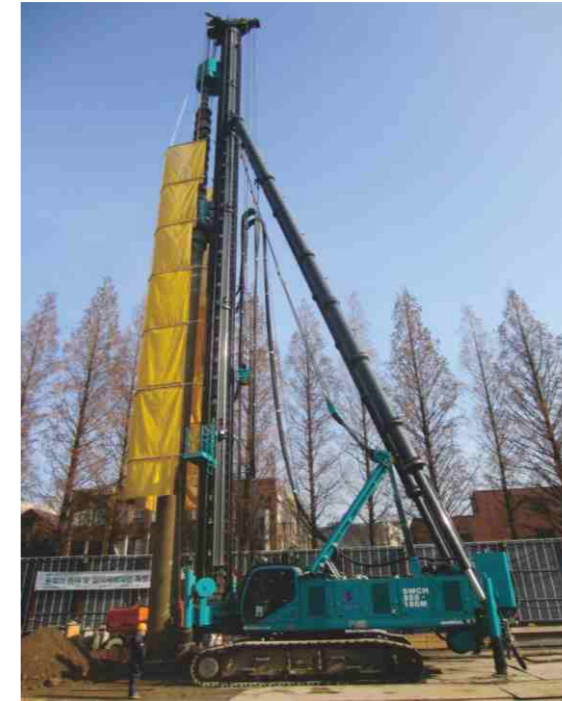
Construction at Hyundai Construction Site in Seoul, South Korea
