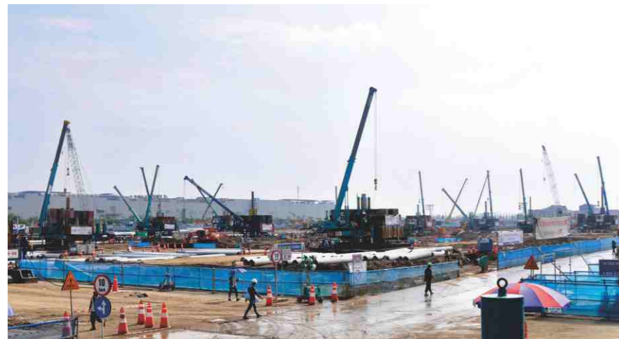
Construction at Samsung Construction Site in Bac Ninh, Vietnam
