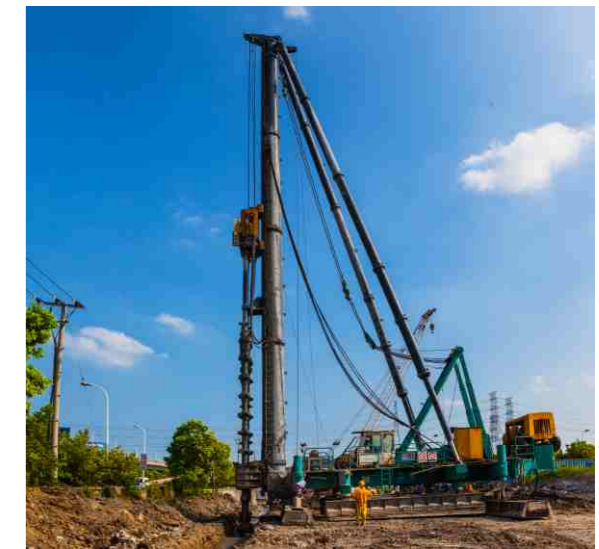
Construction of Three Axis Mixing Pile in Shanghai
