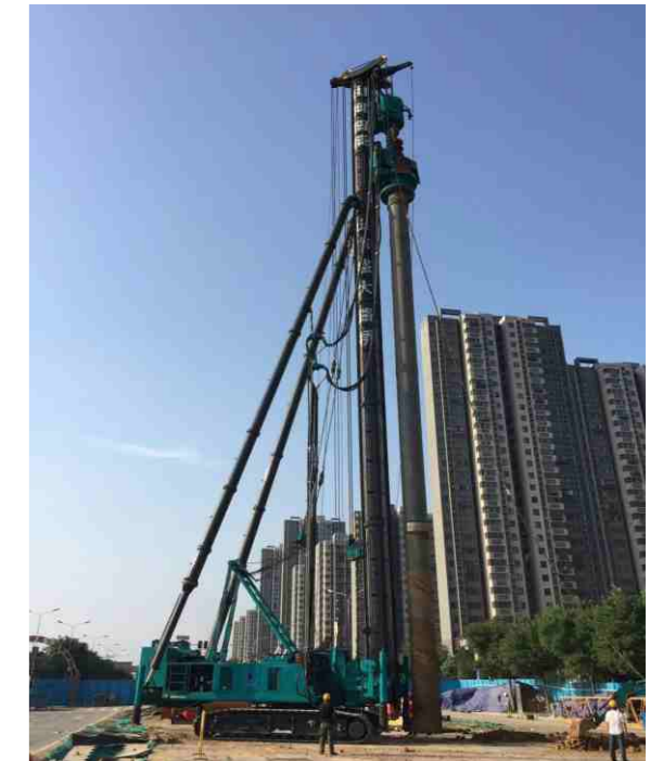
Construction of Jinan Metro
