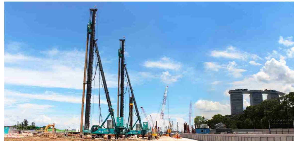
Foundation Construction of Singapore T27 Project
