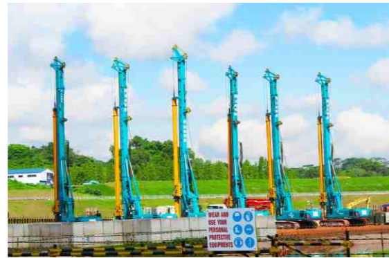
Construction in Singapore
