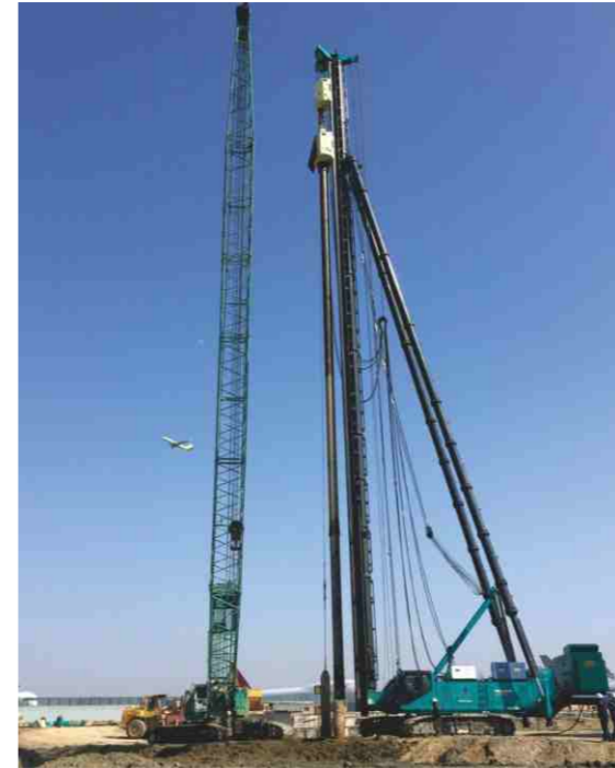
Construction of Asiana Airlines Maintenance Workshop in Yeongjong Island, South Korea
