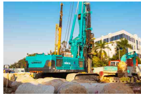
Construction of Xiamen Metro
